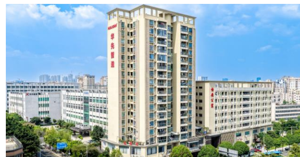
Shenzhen (Tianliao) Digital Intelligence Industrial Park
